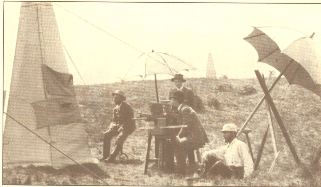
The first torsion balance field measurements (on Ság hill, Transdanubia, Hungary) in 1891. EÖTVÖS can be seen at the telescope
